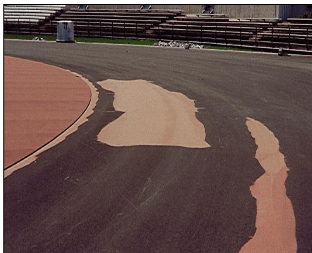
Fig 3. Sub-base after the track surface is ground down.
