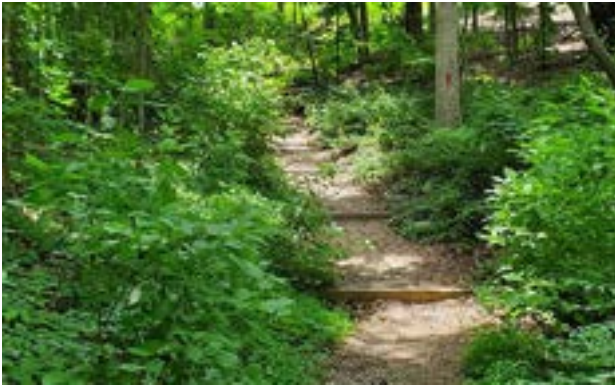
Figure 6-12. Illustration of proposed walking surface supported by tree log steps where necessary. Credit: Elachee Nature Science Center
